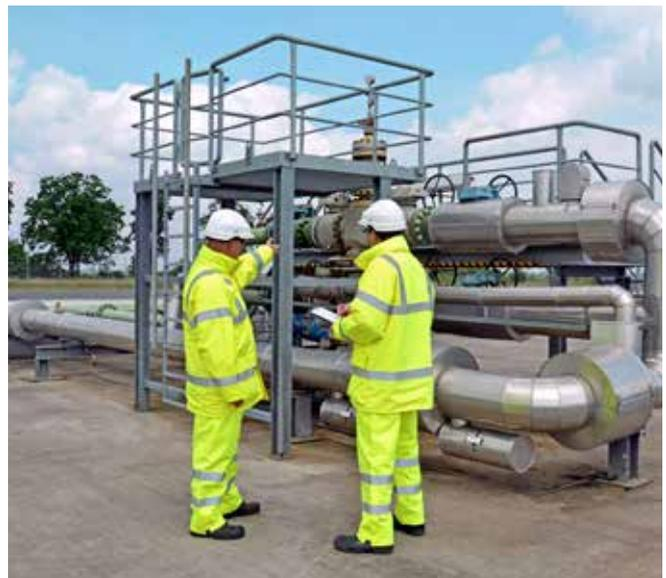
Operational checks at an oil cavern wellhead
